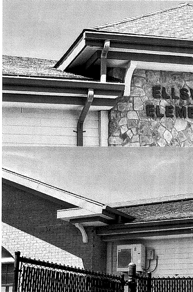
Where the eaves, soffits and fascia return onto the existing roof, the contractor is expected to utilize the same metal panel as the balance of the project. If the conditions don't allow the panel seam to fit, a flat metal panel (by roofing Manufacturer) will be acceptable at these locations. The detail against the stone will be similar to detail P/A530 with a new saw cut reglet/flashng installed.
