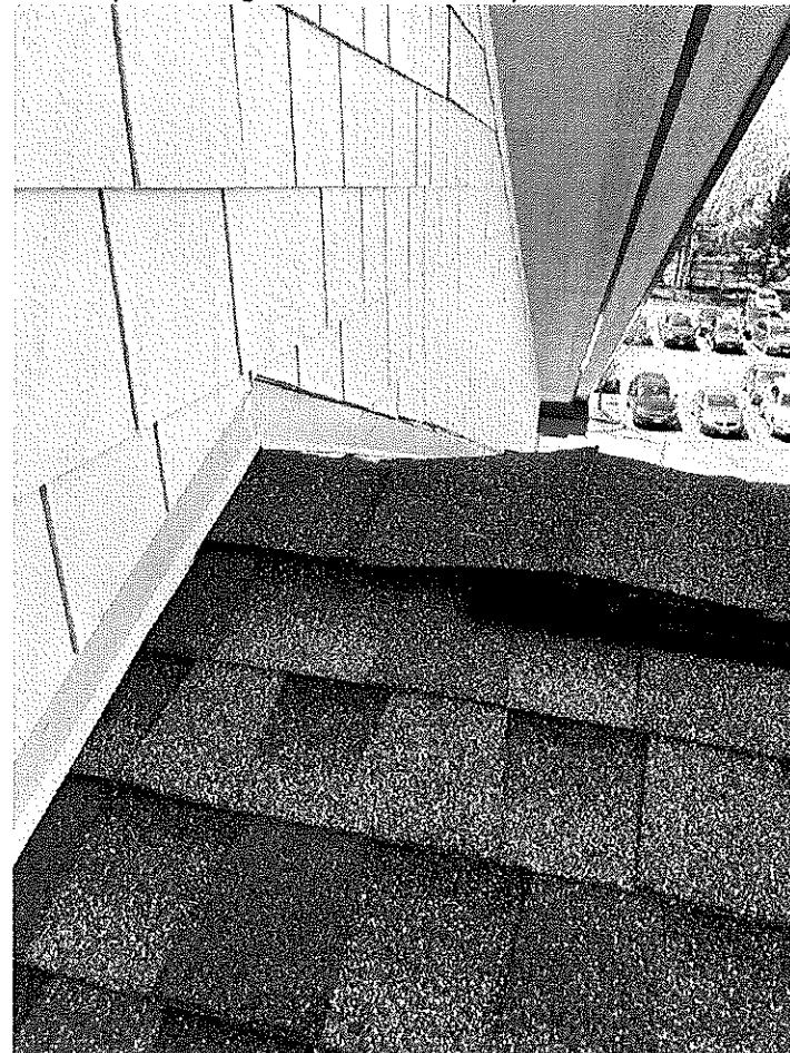
See detail R/A530. Contractor to assume that the shingles may need to be cut/raised/modified to execute this detail. This may include adding additional metal flashing matching existing in kind.
