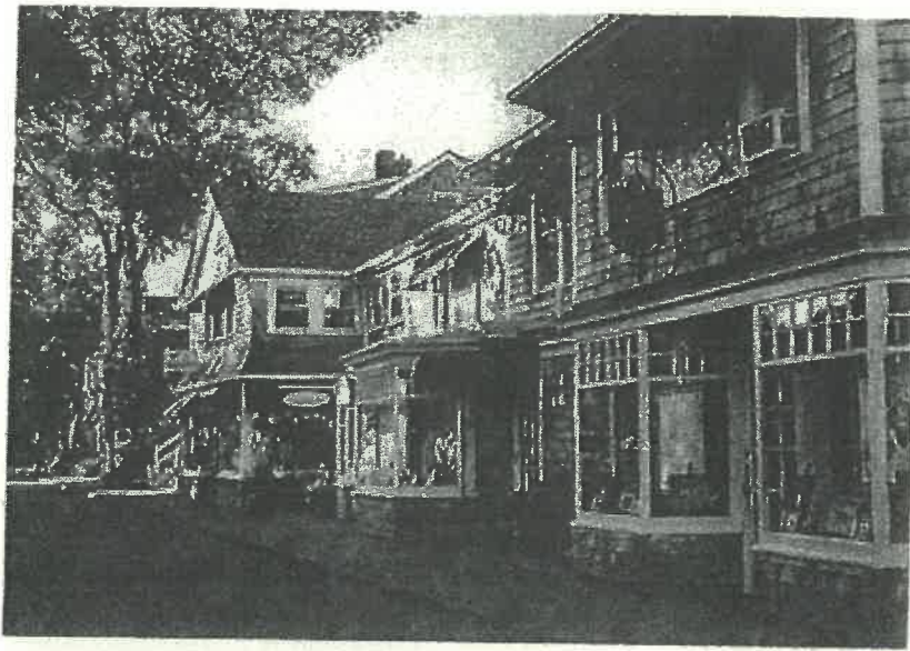
Apts over village shops. Well designed. Walkable.
