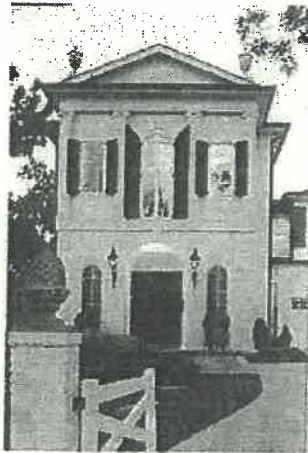
Small carriage house on possible larger property.
